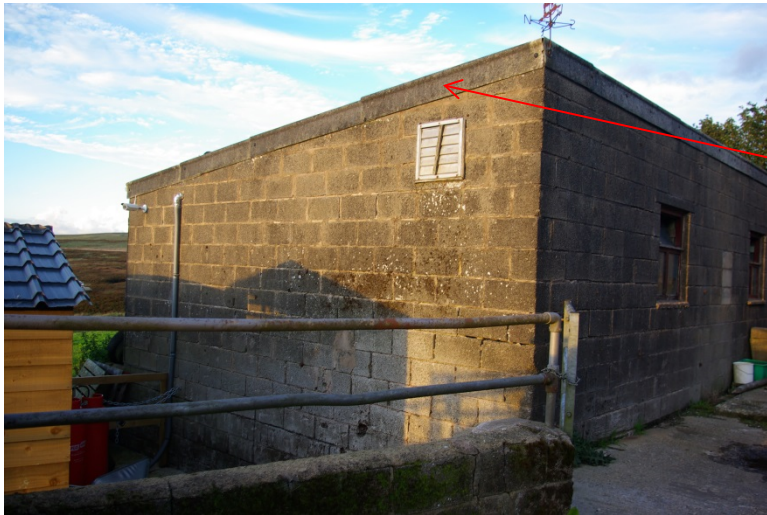
Building 4 Concrete block Capped roof verges
