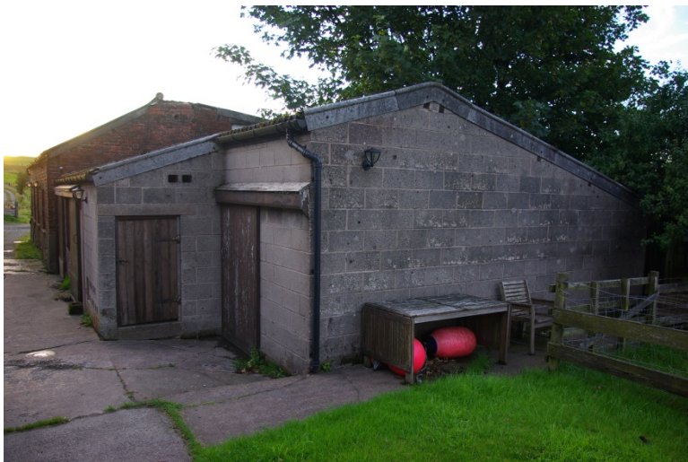
Building 5 - East Concrete block, well sealed
